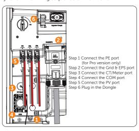
Figure 7-14 Wiring sequence of the inverter
