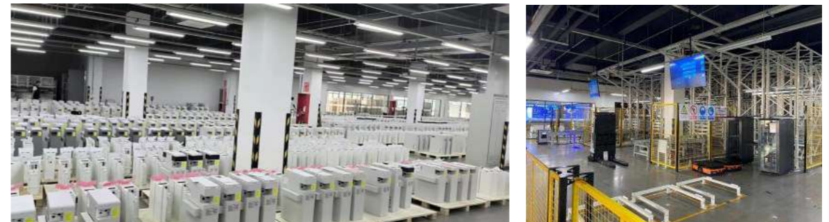
Battery Static Warehouse Racking System Before (Left Figure) and After (Right Figure) Renovation
